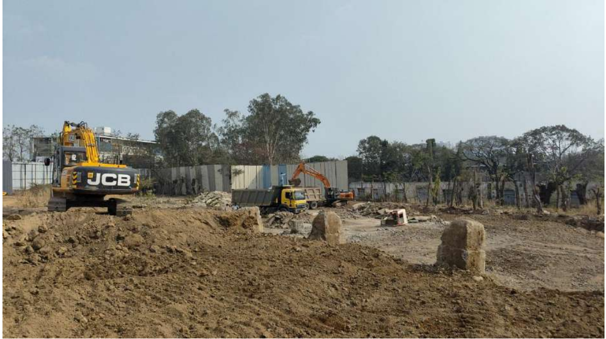
Tower E TOWER E excavation Work In Progress.
