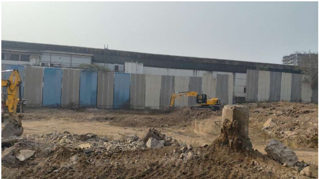
Tower F - TOWER F and G excavation Work In Progress.
